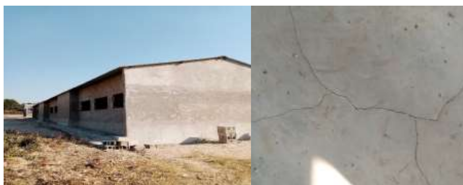
1. Kansanshi Primary School: Complete block and Floor with cracks
