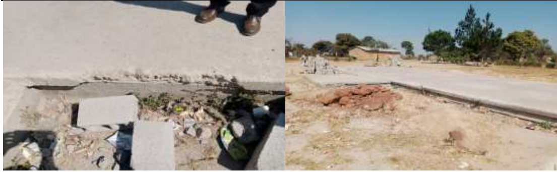
3. IX3 CRB at Mashipi Primary School: Poorly done slab, poor mixture of concrete and no ant guard
