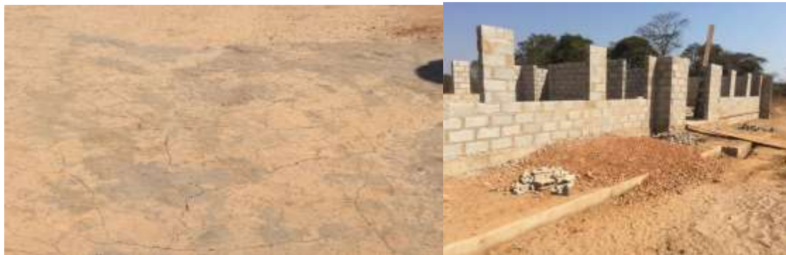
4. IX3 CRB at Mayonde Primary School: Poorly done slab, used gravel for mixture instead of quarry dust.
