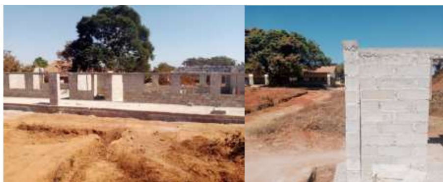
1. CRB at Kimale Secondary School: Thin ream beam and bent pillar
